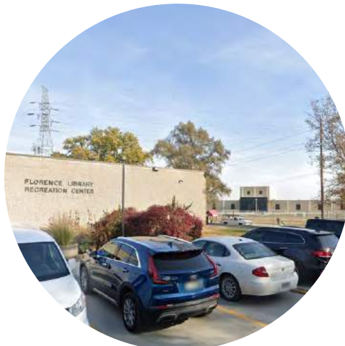
ACCESS TO THE LIBRARY: Community members arrive by bus line 30, private vehicles, or walk.
